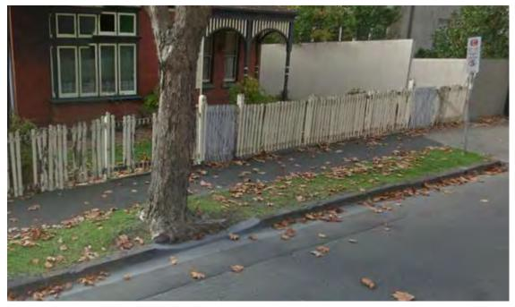
Figure 41: Modified kerb reinstatement method to allow space for buttressing trees roots and maintain effective road drainage (Photo Source: Steve Watt, Stonnington City Council)
