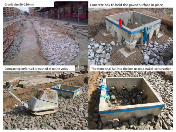
Figure 49: Concrete boxes for tree planting surrounded by the Stockholm structural soil (City of Stockholm)
