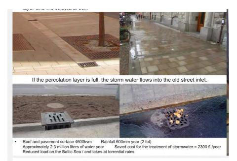
Figure 51: Rainwater runoff from buildings is directed in to the Stockholm structural soil zones for use by the street trees (City of Stockholm)
