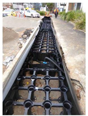
Figure 46: Trench of soil cells prior to the addition of uncompacted soil (Photo Source: Steve Watt, Stonnington City Council)
