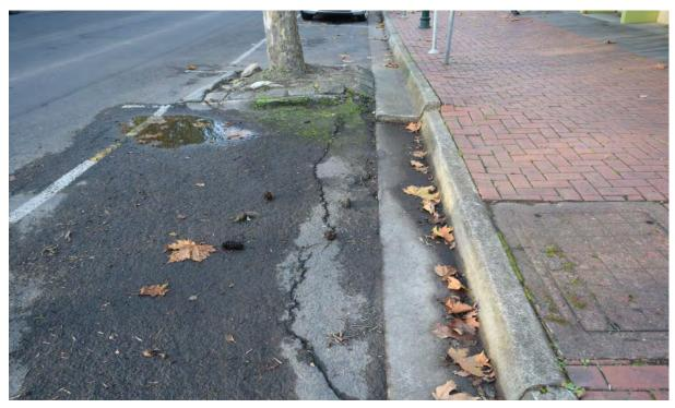
Figure 15: Asphalt cracking presumably in response to surface tree roots
