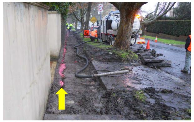
Figure 37: Indicative location (arrow) to install root barrier within footpath, close to private assets (Photo source: Chris Sullivan)
