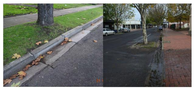
Figure 17: Kerb damage
