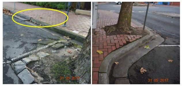
Figure 19: Footpath lifting and asphalt damage presumably in response to root growth
