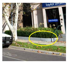
Figure 22: Minor cracking of retaining walls
