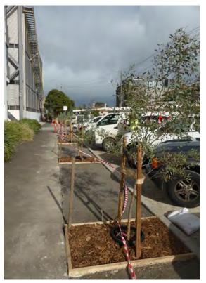
Figure 47: New trees planted in soil cell trench (Photo Source: Steve Watt, Stonnington City Council)
