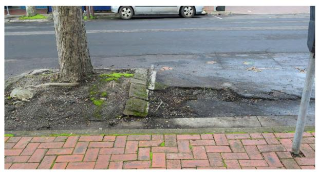
Figure 16: Asphalt damage adjacent to the small tree cut out
